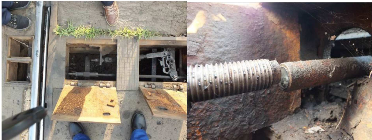
Figure: Fracture of the short pull rod
