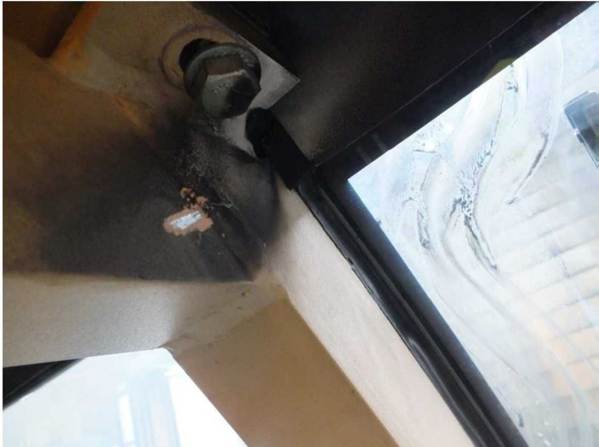
Figure: Marks of an electric arc in the driver's cab
