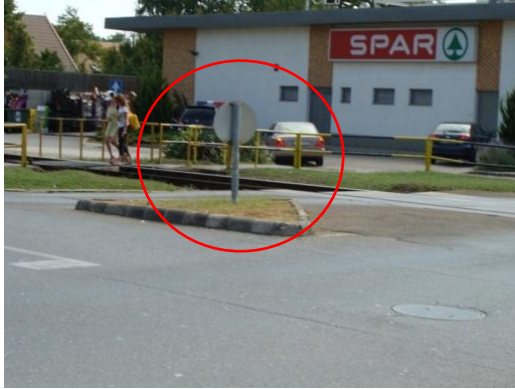
Traffic sign in wrong position
