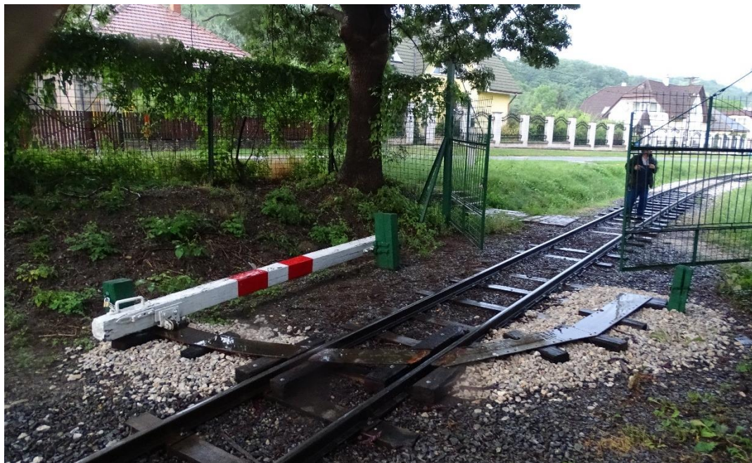
Figure 10: The red-white track barrier and the gate forced open by the runaway wagons, in the morning after the occurrence (the position of the gate leaves in the photo do not reflect the direction of roll of the wagons)
