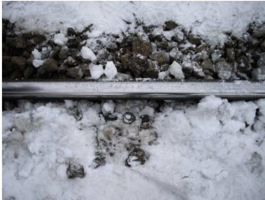
Figure 7: marks of ploughing and corrosion
