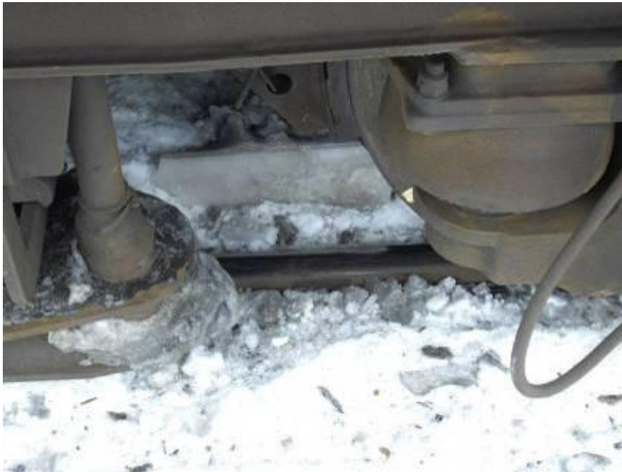
Figure 6: second derailment mark on the rail
