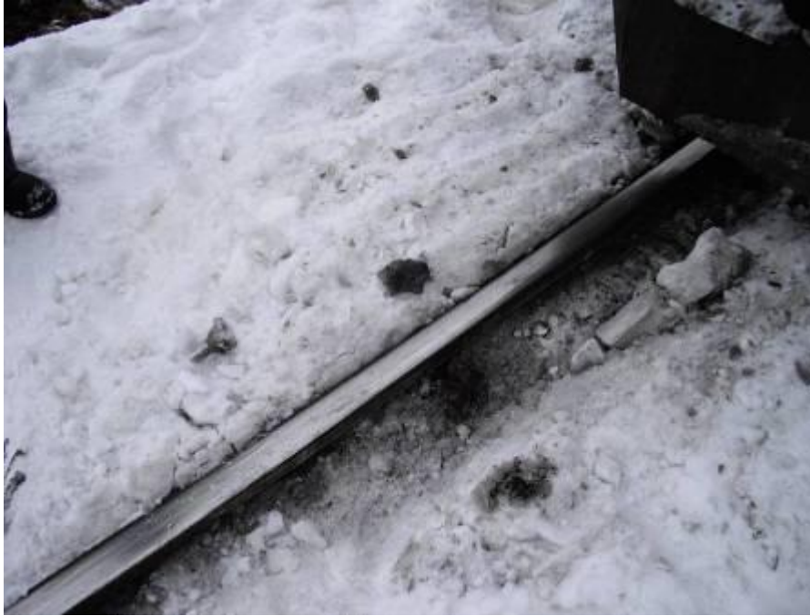
Figure 5: first derailment mark on the rail
