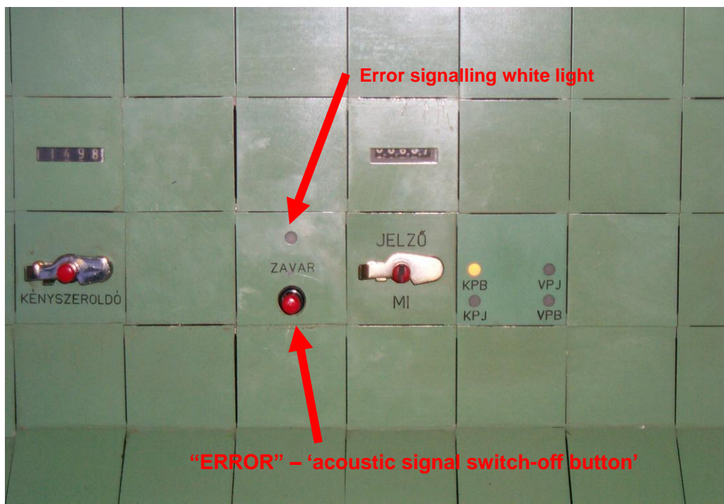
Figure 4: Control panel of Domino 55 type signal box
