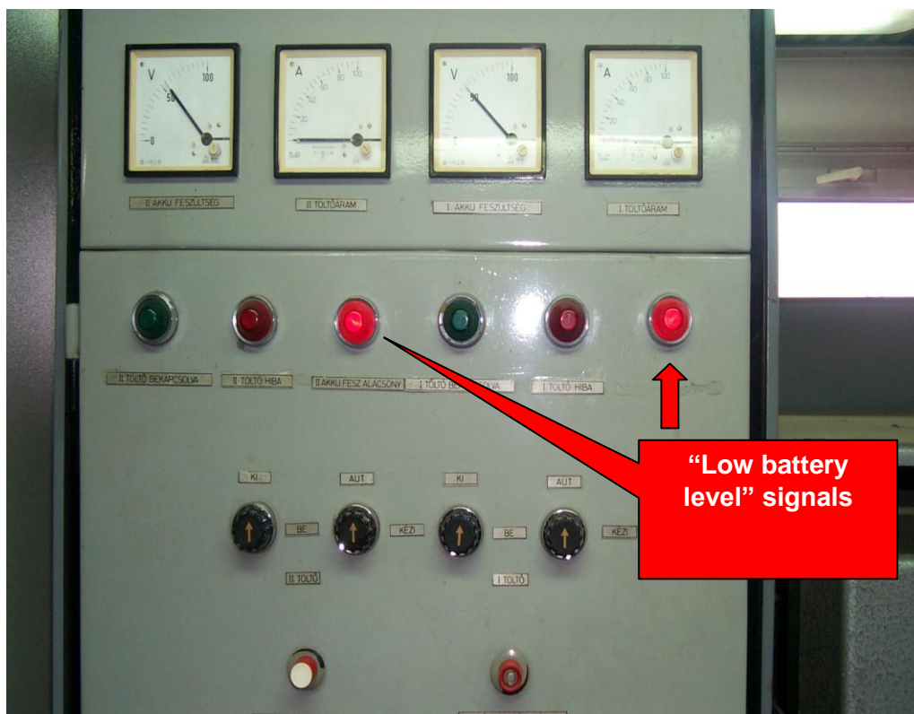
Figure 5: E-11 type battery charger
