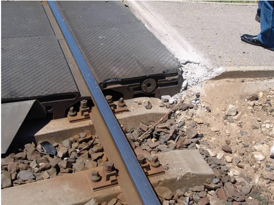
Figure 5: The slightly shifted STRAIL plate at the pedestrian crossing
