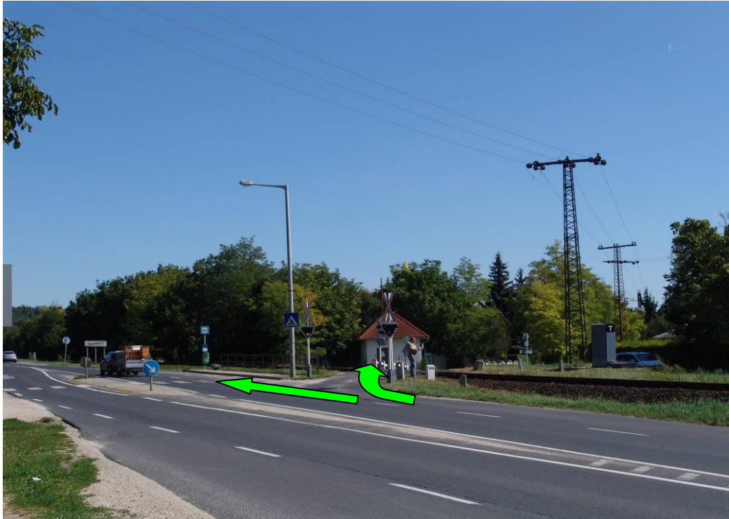
Figure 23: LC no. AS373 secured with warning lights in the direction of Balatonakarattya
