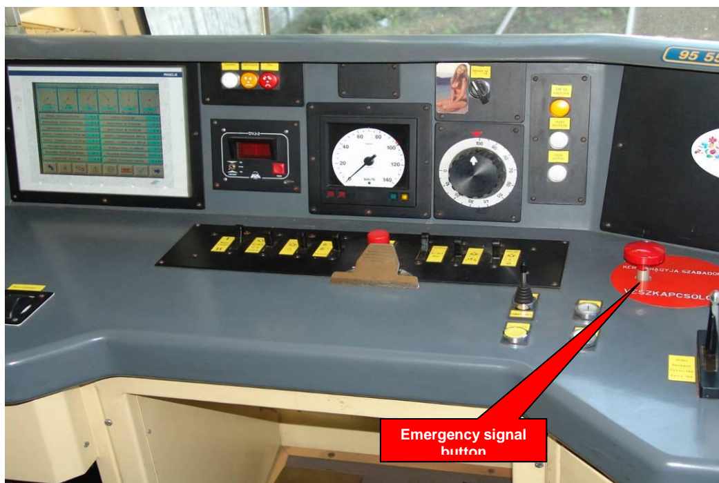
Figure 15: The driver's cab of the locomotive (registration no. M41-2311)
