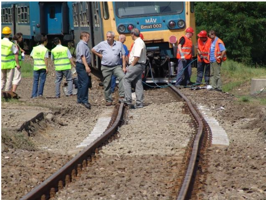
Figure 3: The rail track at the accident site
