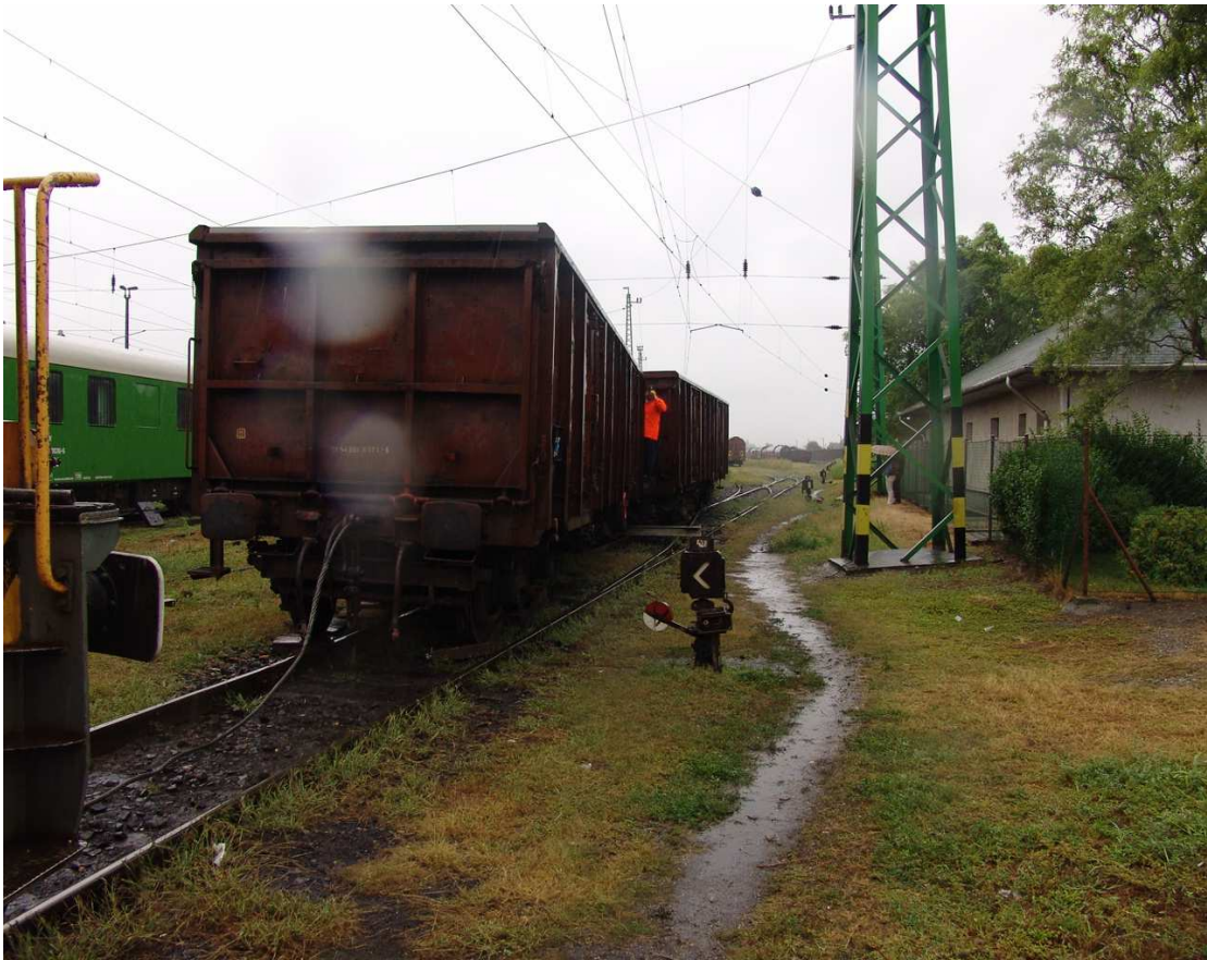
Figure 5: Location of the accident (switches 427, 428)
